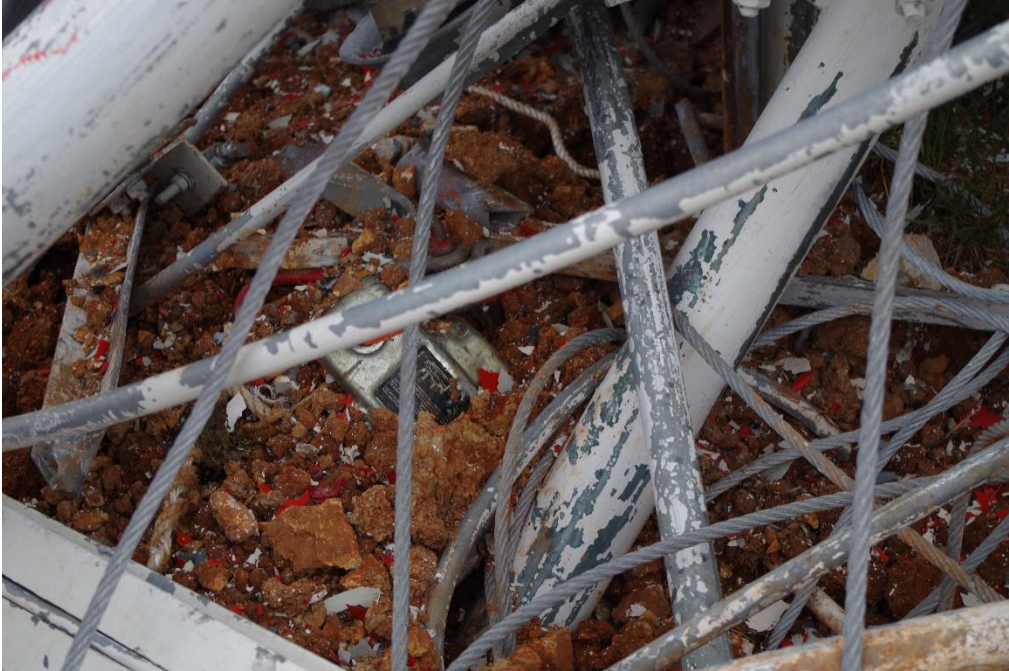
Figure 16. T-532D Come-a-long in Debris
