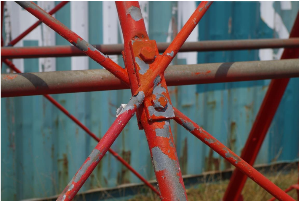
Figure 13. Bolted Connection between Diagonals and Redundant Horizontal
