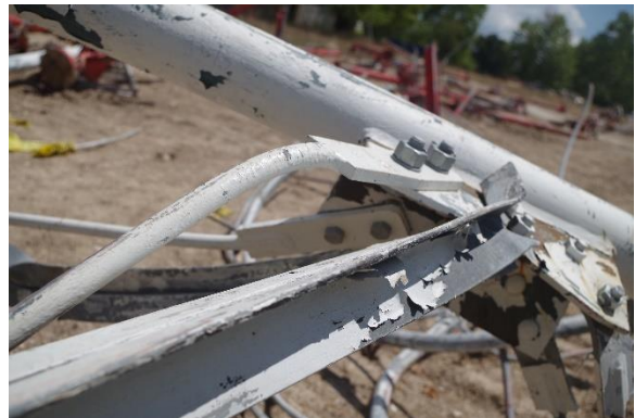
Figure 10. New bolts Installed on Two Diagonals at 100' Tower Elevation
